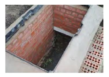
**Temporary works.** After local excavation, we dammed the culvert and conducted over pumping to clear the debris and allow CCTV access. Prioritising safety, we established confined space access with emergency response for operatives to conduct the surveys.
